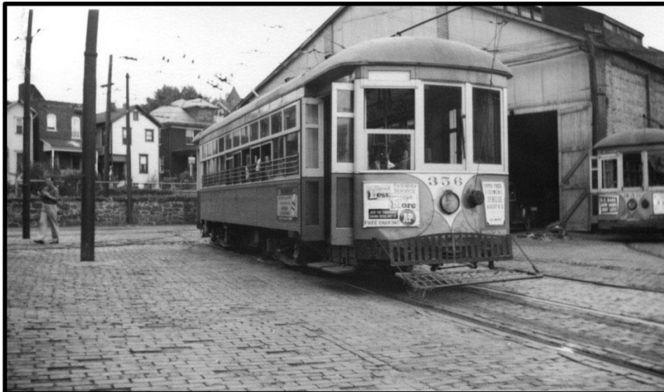
Figure 3. Undated photograph showing trolley exiting the northeast façade of 630 Central Avenue. Note original corrugated metal cladding and original car barn door.
