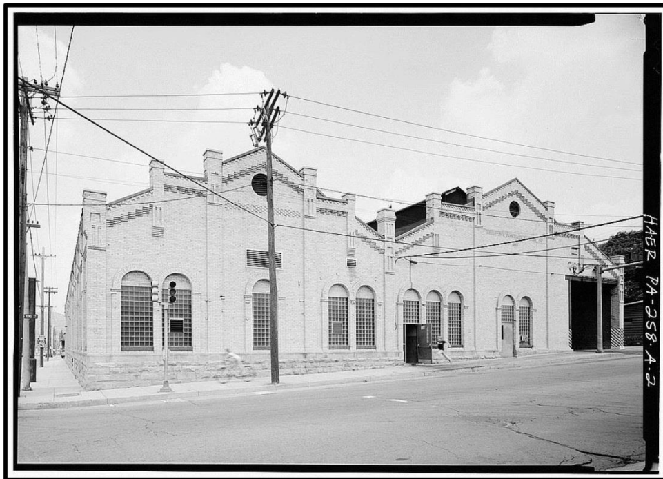
Figure 10. 1991 HABS photograph of Bond Street (southwest) façade of 630 Central Avenue. Note original window and door units have been replaced.
