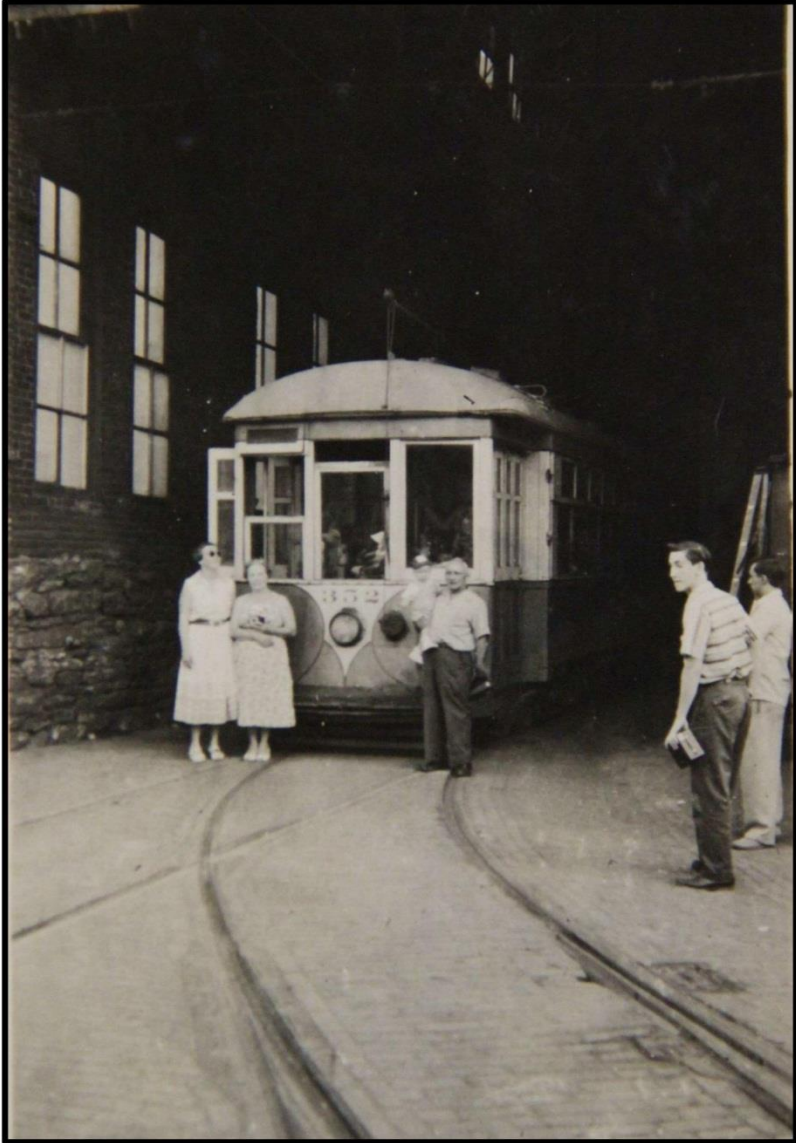
Figure 5. 1961 photograph showing trolley exiting the northeast façade of 630 Central Avenue. Note original four-over-four light, double-hung wood sash windows (left).
