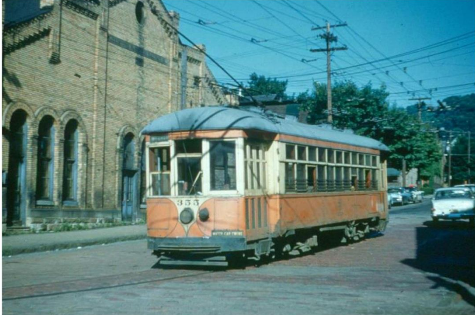
Figure 6. Undated (ca. 1955-64) photograph showing trolley in front of Bond Street (southwest) façade of 630 Central Avenue. Note original window and door units.
