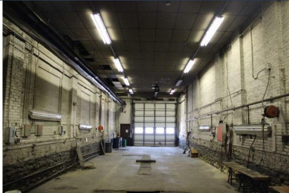
630 Central Avenue, interior, showing long, open work bay area, facing northeast.
