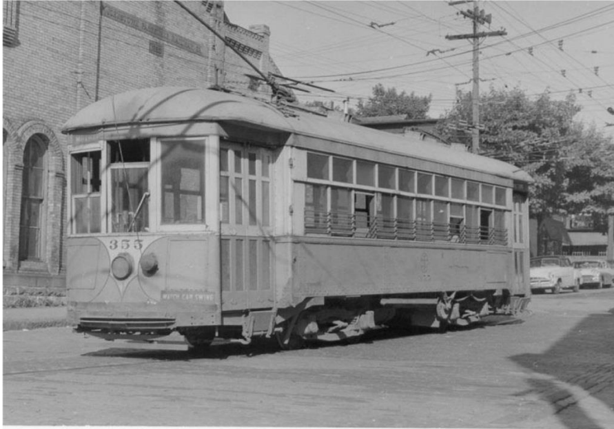
Figure 7. Undated (ca. 1955-64) photograph showing trolley in front of Bond Street (southwest) façade of 630 Central Avenue. Note original window round-headed, four-over-four light, double-hung, wood sash window.
