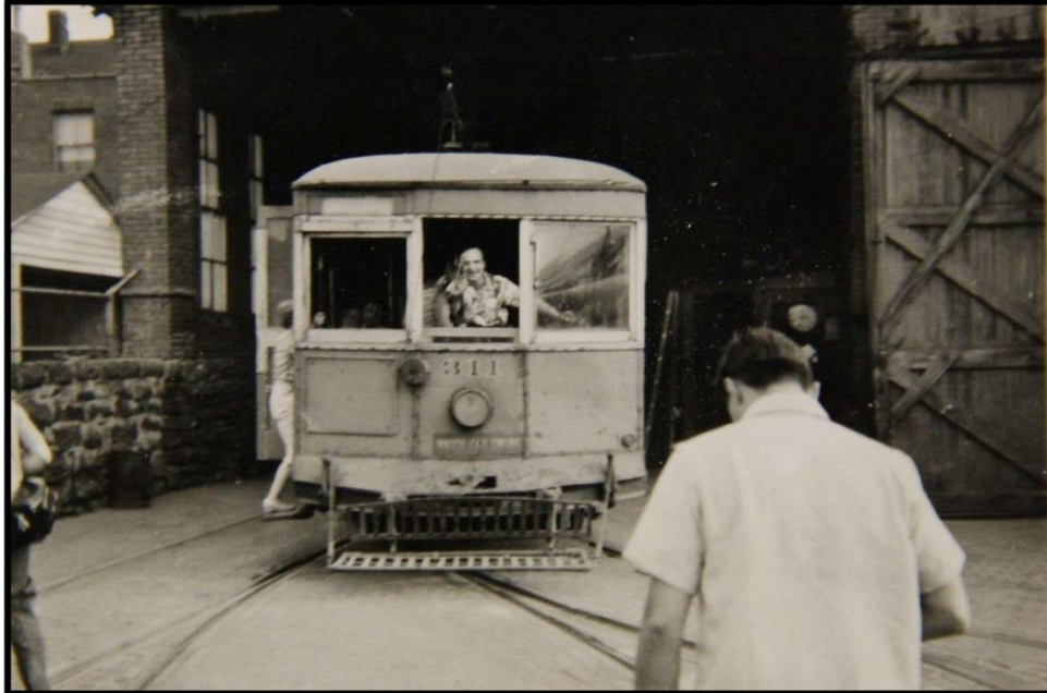
Figure 4. 1961 photograph showing trolley exiting the northeast façade of 630 Central Avenue. Note original four-over-four light, double-hung wood sash windows (left) and original cross-buck car ban doors.
