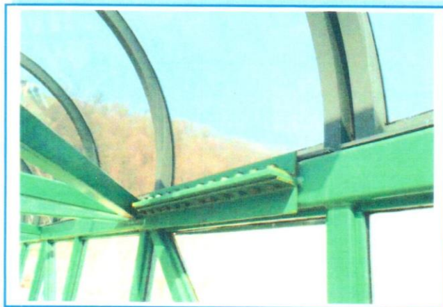
PHOTO 38: Welded and Bolted Splice of the Top Chord at Mid-Span
