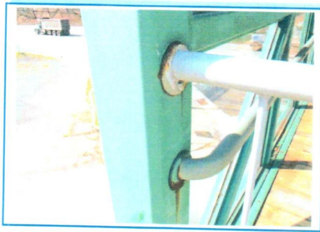
PHOTO 35: Typical Hand Rail to Truss Connection at Portals
