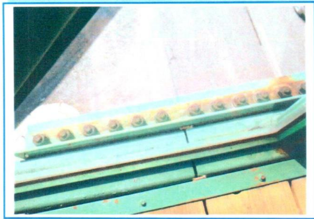
PHOTO 41: Splice to the Bottom Chord
