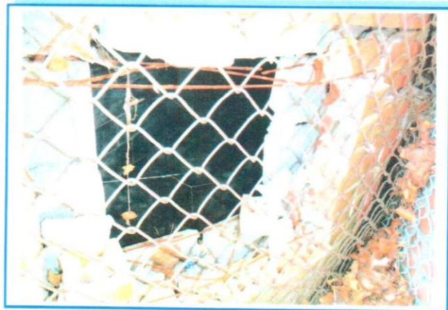
PHOTO 68: 2' Wide x 2' High Hole in Brick Veneer and Concrete Blocks
