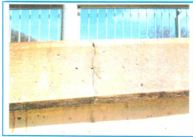
PHOTO 21: Cracking Propagating to Outside Face of Deck
