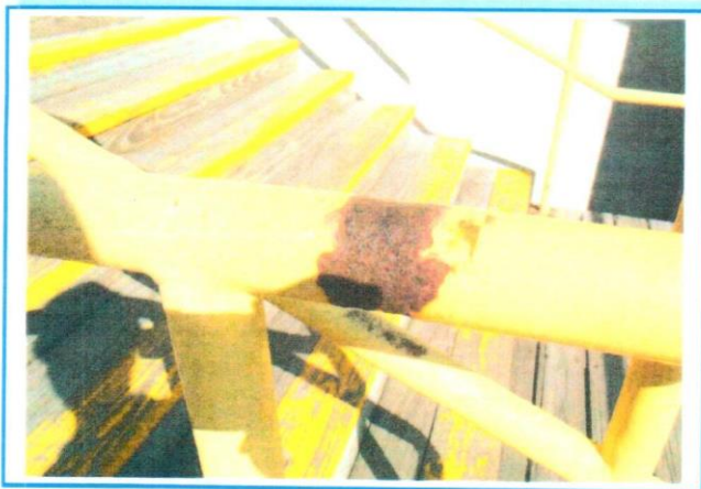
PHOTO 12: Typical Surface Rust and Section Loss at Random Locations of the Hand Railing at the West Side Stairs
