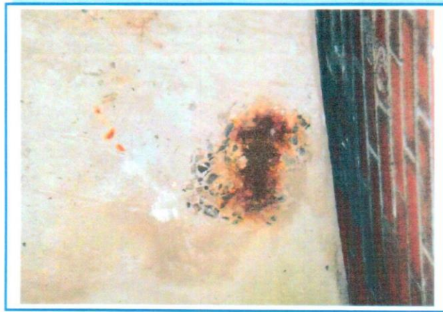
PHOTO 83: Spall 4" Long x 3" Wide x 1" deep with Exposed and Rusted Rebar Pier Cap 3
