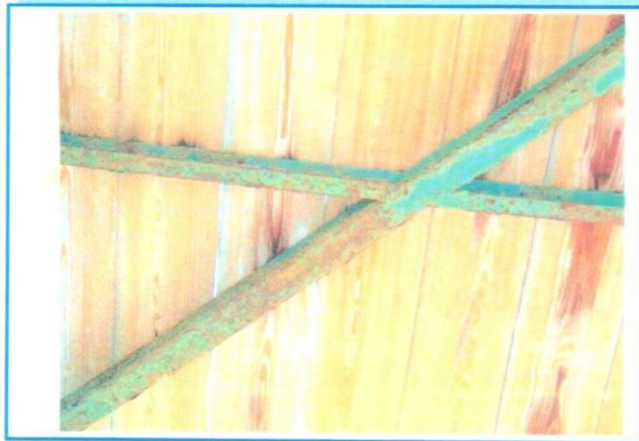
PHOTO 48: Typical Surface Rust to the Cross Member and Stinger Channel
