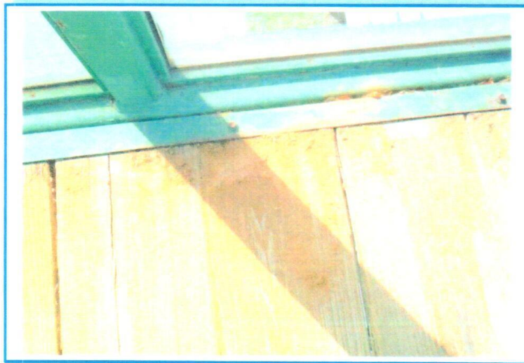
PHOTO 32: Dry Rot to Deck Planks throughout
