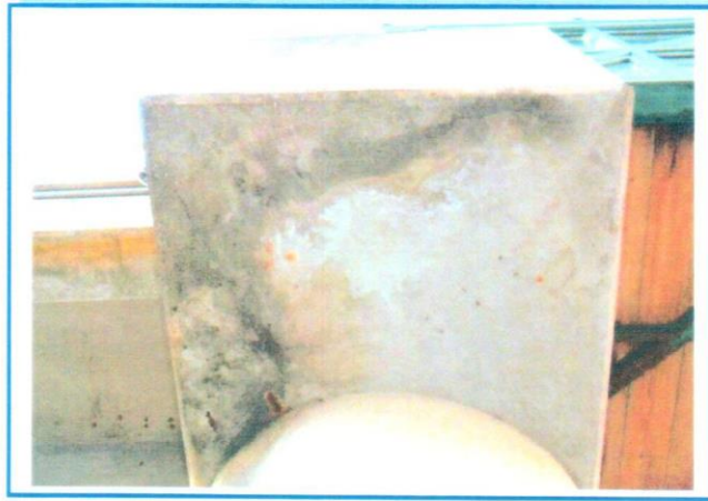
PHOTO 75: General Condition of Pier Cap 2 – Exposed Chairs
