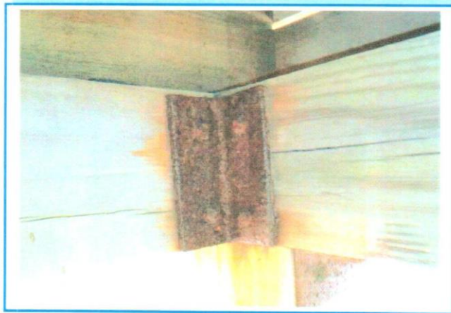
PHOTO 16: Typical Rust and Section Loss to Angles and Bolts at the Connections of the West Side Landings and Stairs
