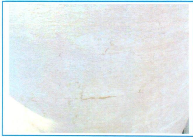
PHOTO 77: Hairline Map Cracking to Pier 2 Face
