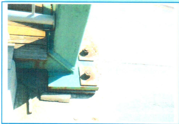
PHOTO 28: West Right Truss Bearing – Missing Grout
