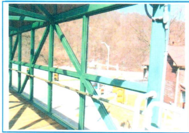
PHOTO 37: Typical Welded Connections of the Truss Members
