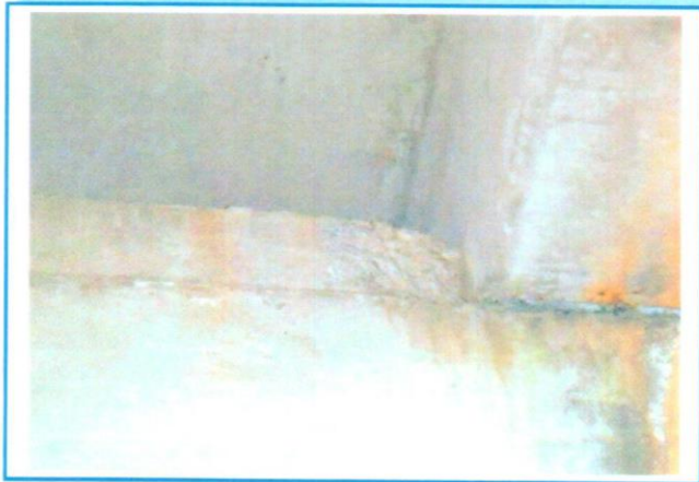
PHOTO 80: Spalling to the Diaphragm above Pier 2
