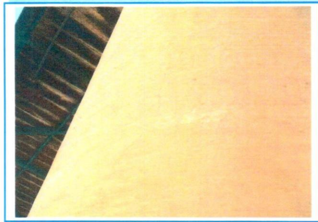
PHOTO 73: Hairline Cracking to Face of Pier 1
