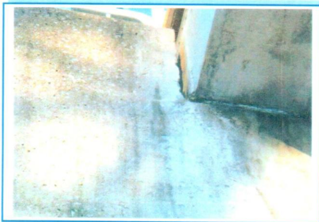
PHOTO 76: Hairline Cracking to Pier Cap 2
