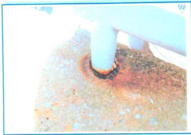
PHOTO 63: 100% Section Loss to the First Post of Second Hand Railing of the Top Ramp
