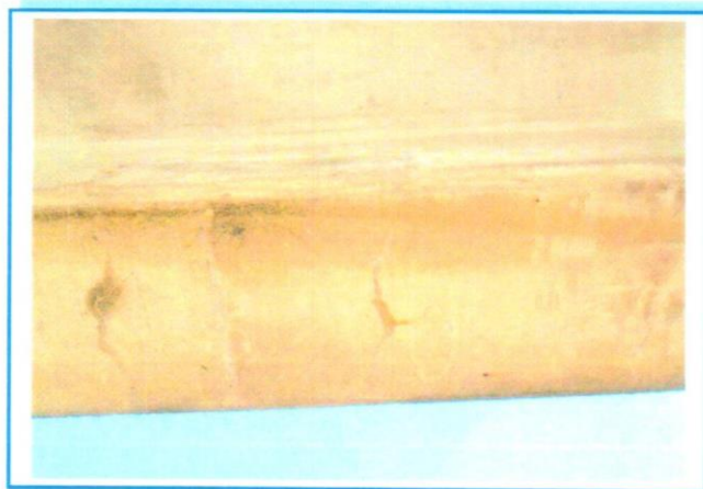
PHOTO 86: Hairline Cracking to Each Girder of Span 3 Propagates from Outside Faces
