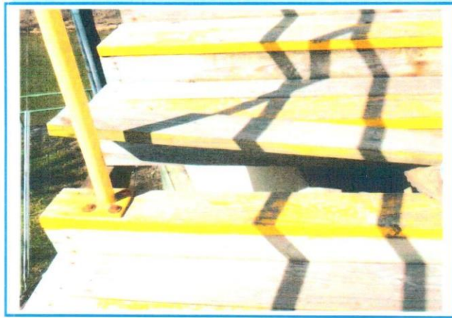
PHOTO 9: Unsecure Tread Board, Step 5, 3 rd Stairs, West Side Stairs
