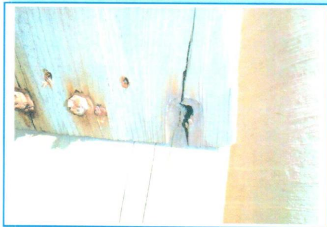
PHOTO 18: Missing Bolt at Knee Bracing of the West Side Landings, Typical Throughout
