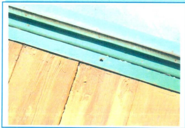
PHOTO 42: Missing Bolt at Deck Angle
