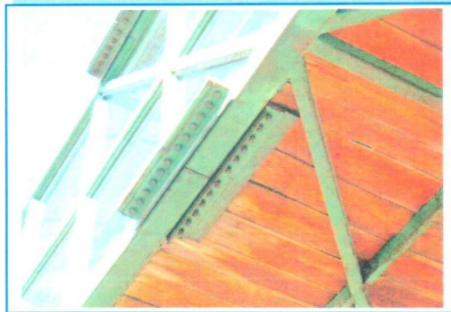
PHOTO 50: General Condition of the Bottom Chord Splice at Mid-Span
