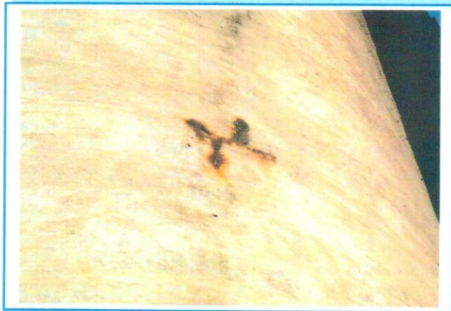
PHOTO 72: Minimum Cover of Reinforcement at Pier 1
