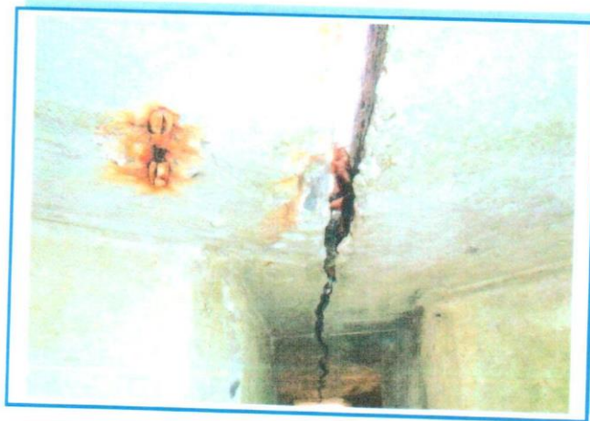
PHOTO 100: Missing Joint Material in Deck over Pier 5
