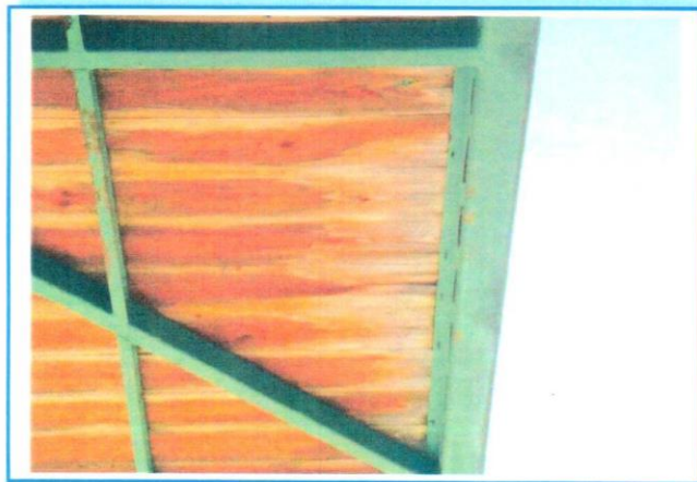
PHOTO 46: Dry Rot to the Outside Edges of the Underside of Deck
