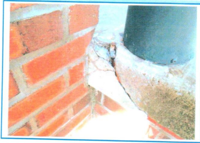
PHOTO 57: Diagonal Crack with Delamination to the First Slab of the Left Side of Ramp 6
