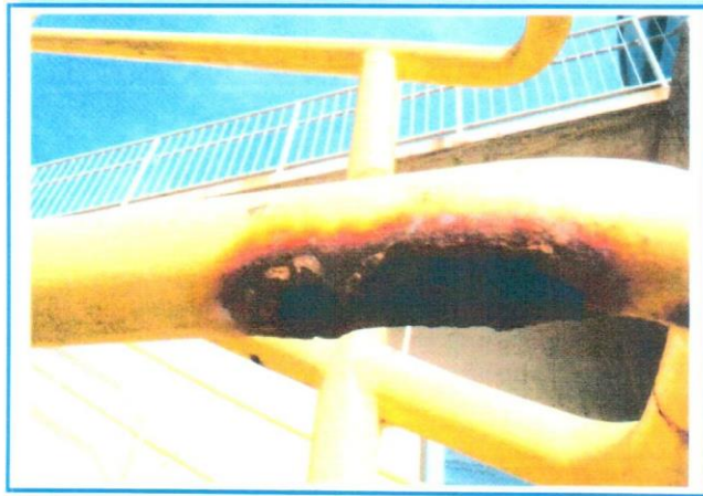
PHOTO 13: 6" long x Full Width Corrosion Hole in Left Side Hand Railing at the Bottom Landing of the West Side Stairs
