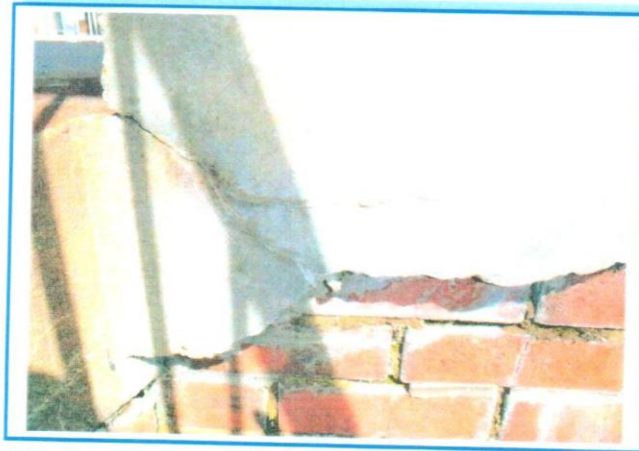
PHOTO 60: Stress Crack to the Left Side of the Bottom step of the Top East Side Stairs
