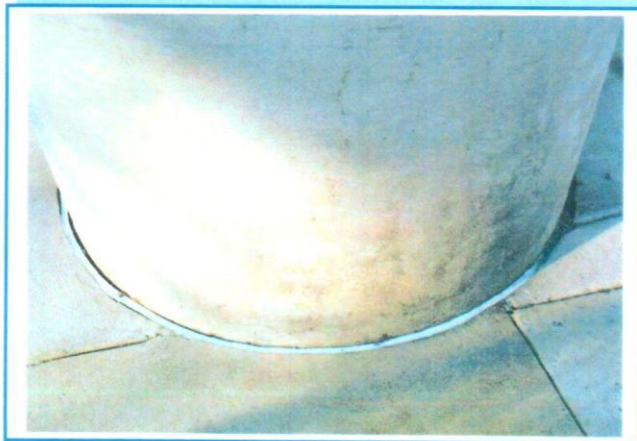
PHOTO 78: Deterioration of the Joint Material at the Base of Pier 2
