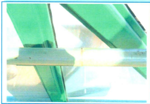
PHOTO 34: Offset to Splice of Hand Rail Typical at most Splices
