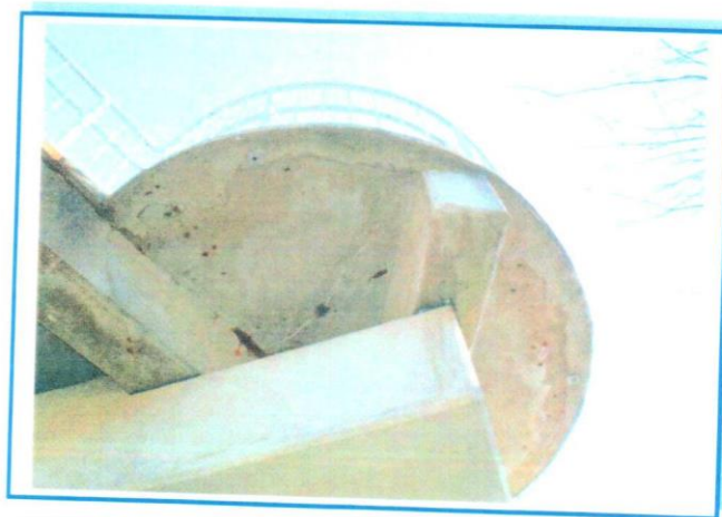
PHOTO 88: General Condition of Deck Underside over Pier 3 (Note: Crack with Efflorescence is also visible on Top)
