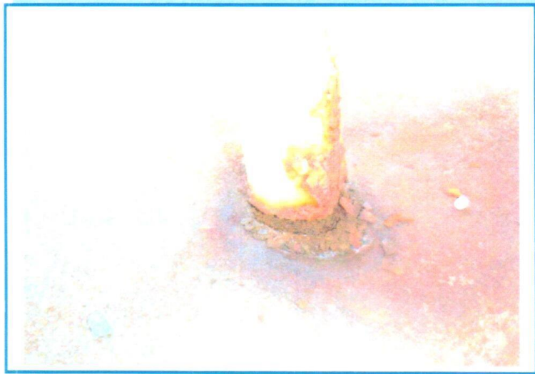
PHOTO 25: 100% Section Loss to the Last Three Post on the Left Side of the West Side Ramp
