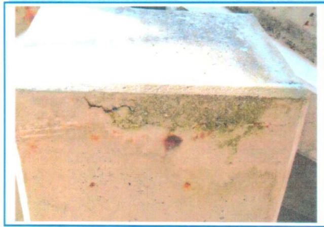
PHOTO 97: Crack with Delamination to Pier Cap 5
