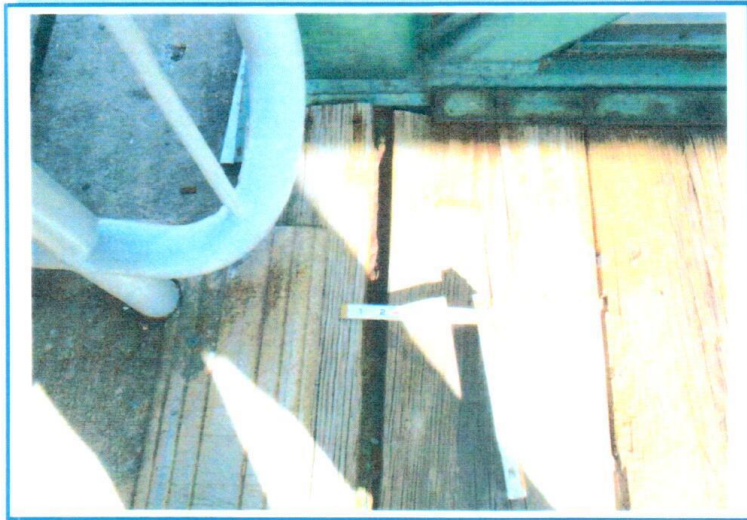
PHOTO 31: 1" Gap between the First and Second Board at the West Side of the Pedestrian Crosswalk
