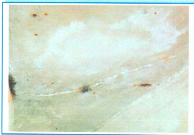
PHOTO 94: Efflorescence Staining and Cracking to the Underside of Deck Typical in Spans 2 through 5
