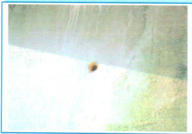
PHOTO 92: Pop Out to Pier Cap 4 with Rust Staining
