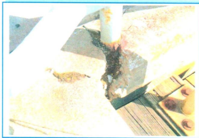
PHOTO 22: Spall Full Height x 4" Wide x 3" Deep Causing Loss of Support to First Post on Right Side of West Ramp Note: Heavy Section Loss to Post
