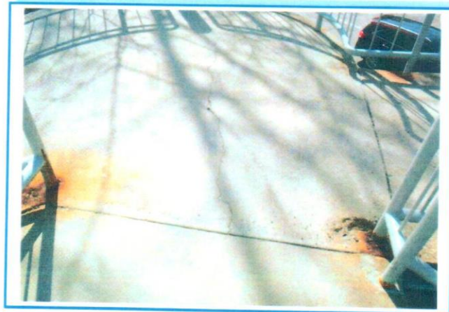
PHOTO 54: Through Crack above Pier 3
