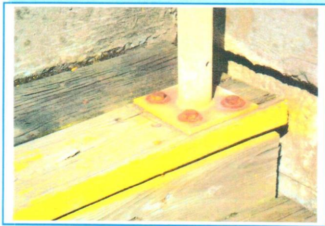
PHOTO 10: Warped Tread Board at the Top of Stairs 3, West Side Stairs
