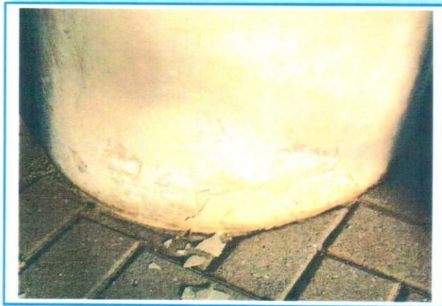
PHOTO 84: Concrete Scaling to Face of Pier 3
