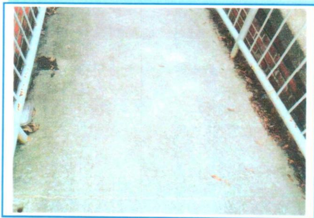
PHOTO 56: Transverse Cracking in Ramp 7 (Note: every 3 to 4 feet)
