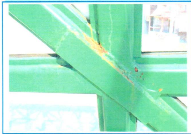
PHOTO 39: Welded Splice to the Intermediate Truss Members
