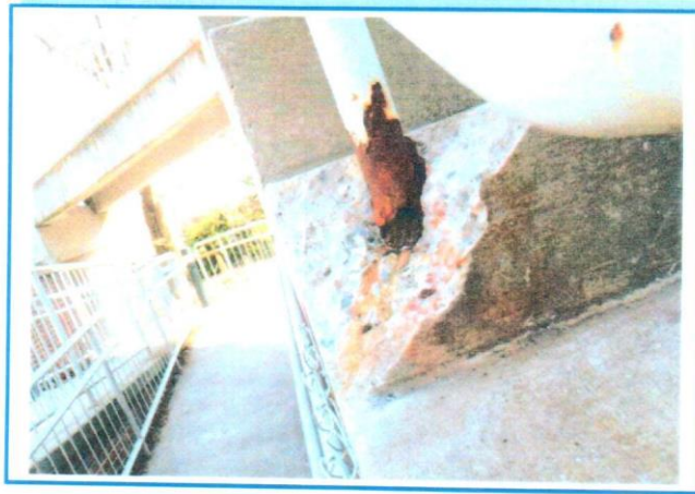
PHOTO 59: Spall in Bottom Step of the Top East Stairs at Middle, Right Side Landing, (Note: Post has 100% Section Loss with corrosion hole)
