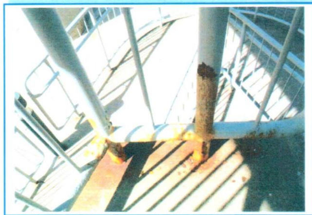
PHOTO 62: Flaking Paint and Surface Rust at Various Locations of the East Side Hand Railing
