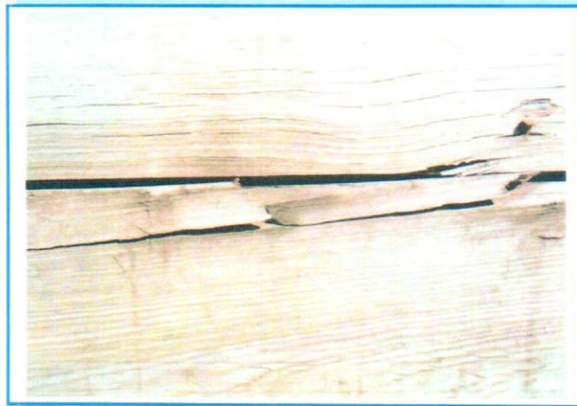
PHOTO 17: Typical Checks and Splits to Timber of the West Side Stairs and Landings
