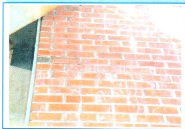
PHOTO 66: Cracking in Brick Veneer and Mortar at Random Locations
